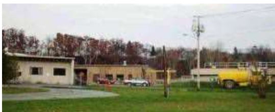
Newport City's wastewater treatment plant. (Courtesy Photo)
